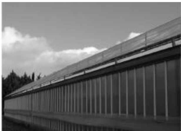
Fig. 9 - Shading and anti hail system running over the roof of a glass greenhouse in southern Italy.
