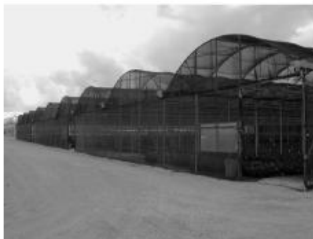
Fig. 10- Steel made vaulted roof with eaves shading structure in central Italy.
