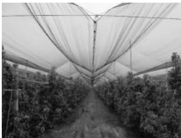
Fig. 7 - Orchard anti hail netting on concrete structure in northern Italy.
