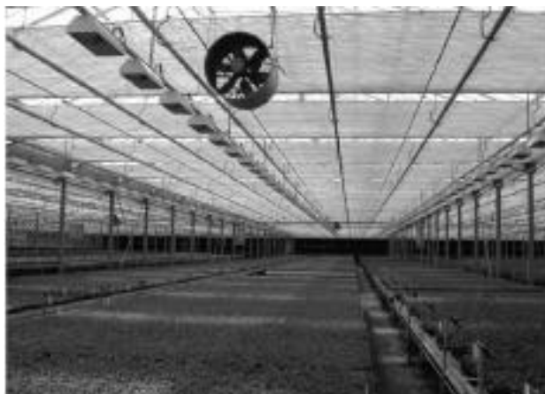
Fig. 12- Thermal and shading screens inside a greenhouse in northern Europe.
