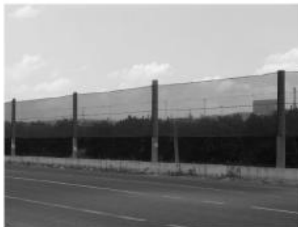
Fig. 6 - Windbreak net supported by a concrete structure in southern Italy.
