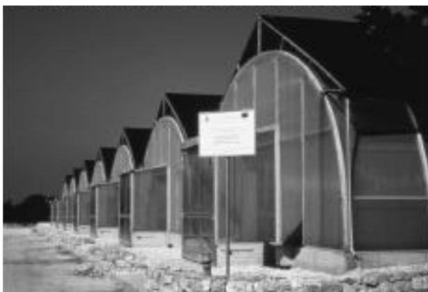
Fig. 14- Screenhouses for certified crop production with a double layer of anti insect nets on the arches and with a stand-alone structure for the shading system at the University of Bari (It).
