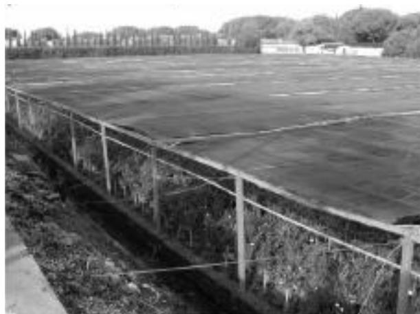
Fig. 11 - Steel made flat roof shading structure in central Italy.
