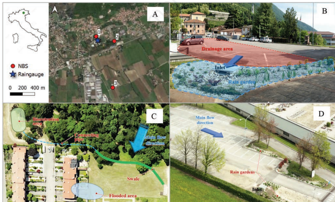
Figure 1. Aerial overview of the study area with location of the investigated nature based solutions (NBSs) (A) and photos of the investigated structures: Libertà Square (B), Grumo Hill (C), and Prati Street (D) (Santorso, IT).
