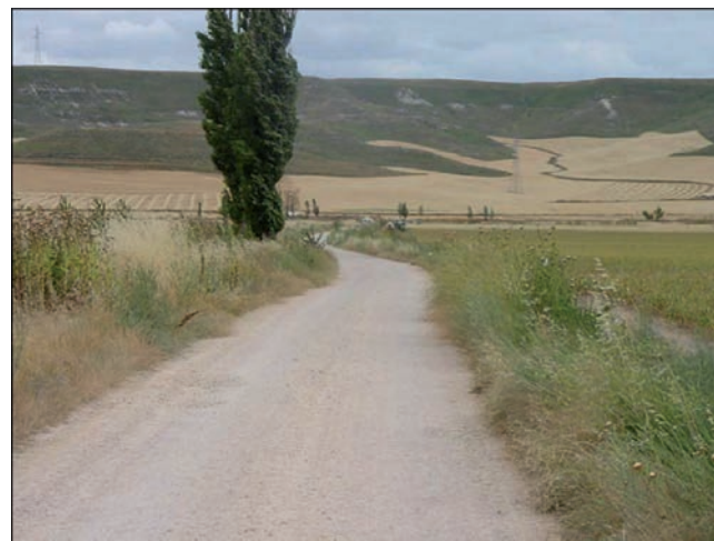
Figure 3. Low volume road paved with macadam.
