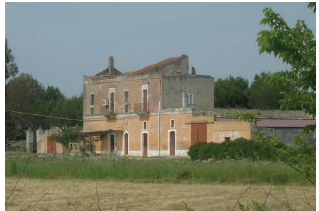
Figure 3. A unitary hilly form of Masseria in the province of Matera.
