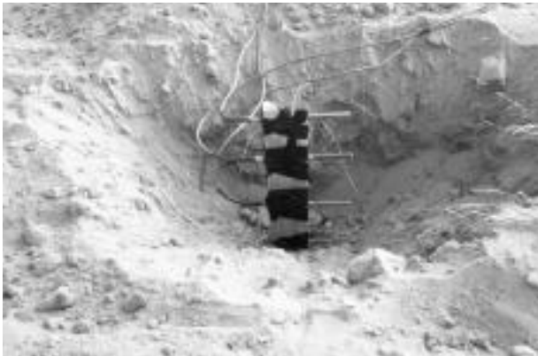
Fig. 2 - Column of Pt 100 probes.
