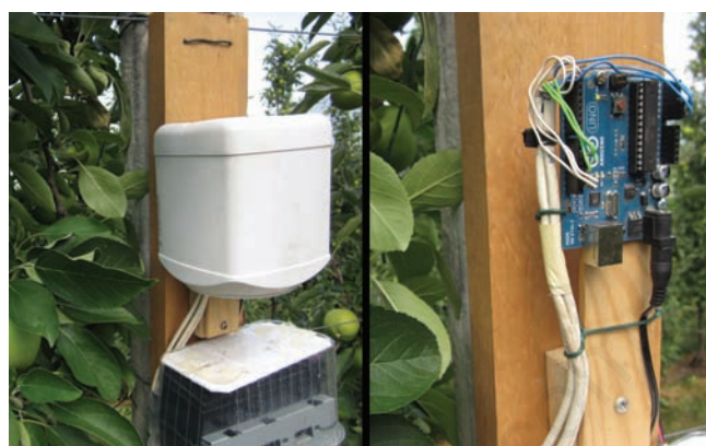
Figure 7. Detail of the tensiometer station shown in Figure 5, displaying the Arduino Uno board and battery with (left) and the Arduino board without (right) protective cover. The cables on the left lead to 3 tensiometers; the black cable on the right side connects to the 12V battery.
