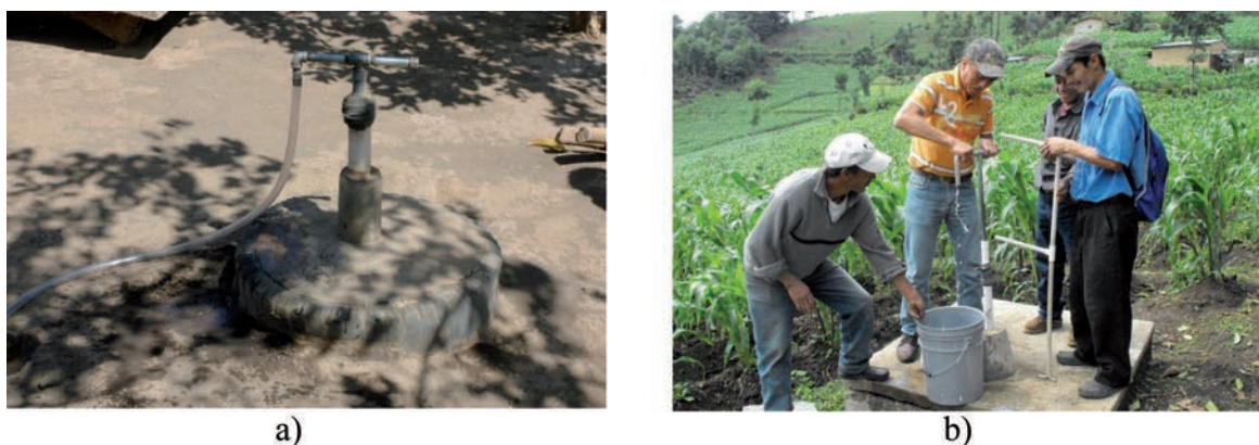
Figure 2. a) The EMAS pump in a drilled well. 2b) Performing analysis on the EMAS pump in an existing well tank.
