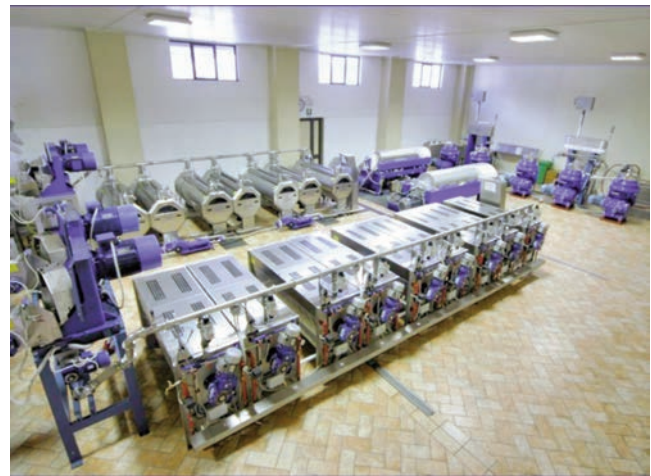
Figure 1. VOO extraction plant equipped with plural malaxing machines in parallel (Photography courtesy Alfa Laval Olive Oil S.p.A.).
